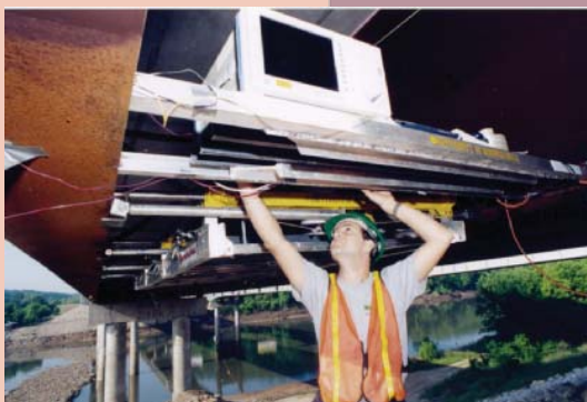
Right: Installation of Fiber Optics on Steel Girders
