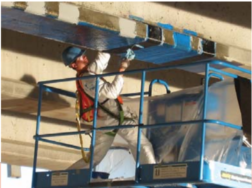
Left: Application of Externally Bonded Composite Reinforcement
