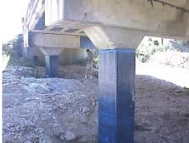
Figure 3: Bridge after column and deck strengthening
