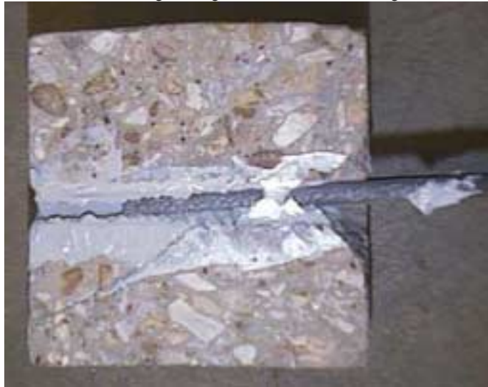
Figure 7: Failure in Bar-Epoxy Interface
