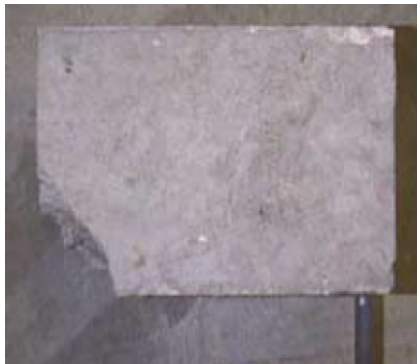
Figure 6: Failure in Concrete
