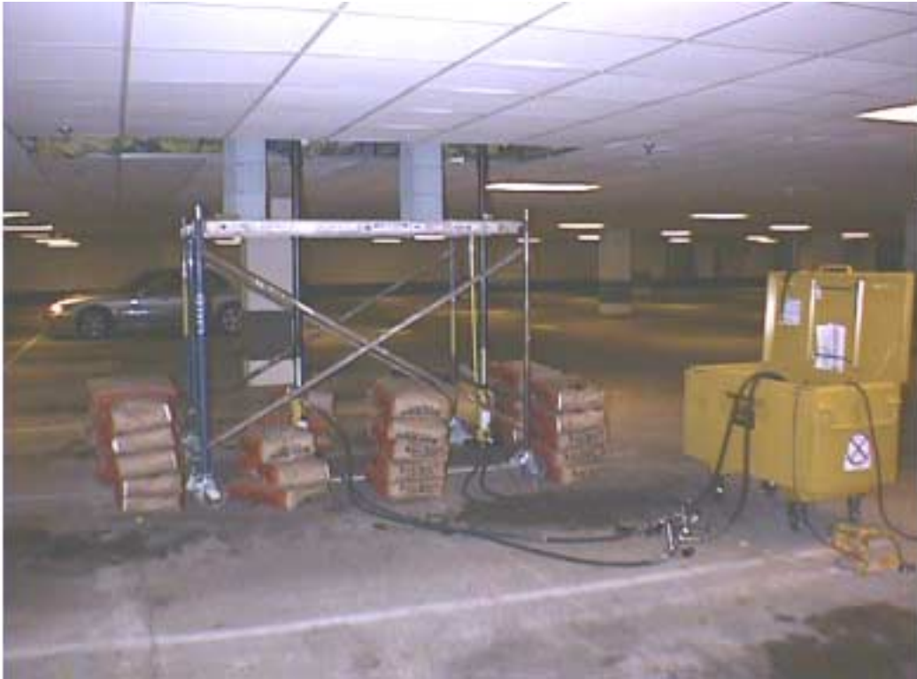
Figure 1: Photograph of hydraulic loading system used by UMR
