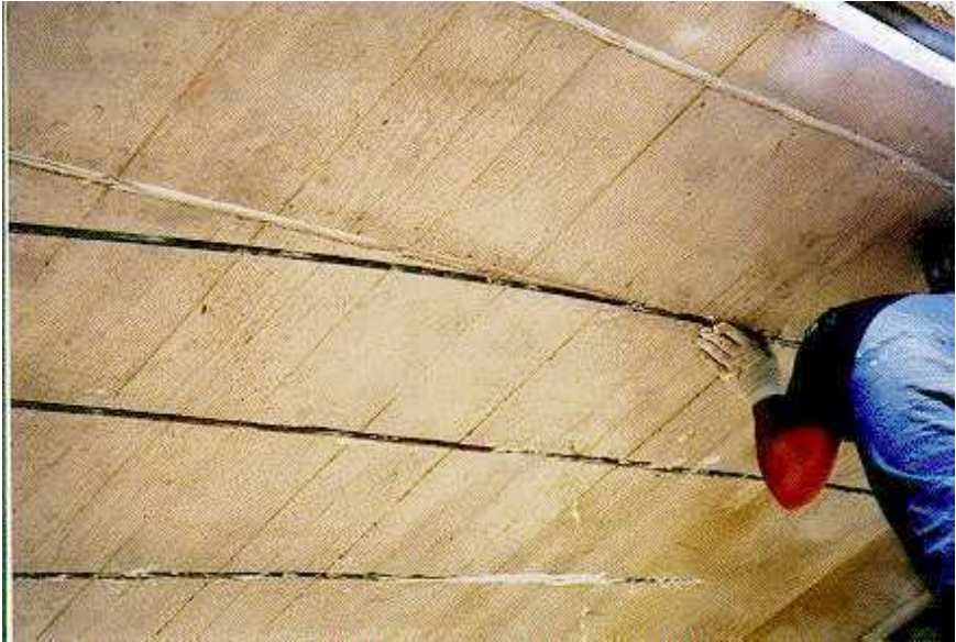
Figure 2. Mounting the NSM FRP rods on bridge deck soffit.
